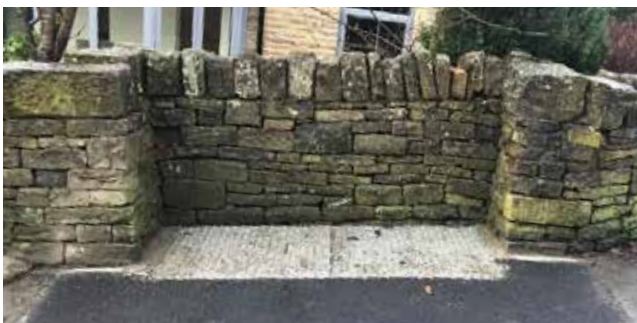
Bespoke cover installation
