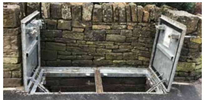
Covers incorporate seals and recessed padlock facility
